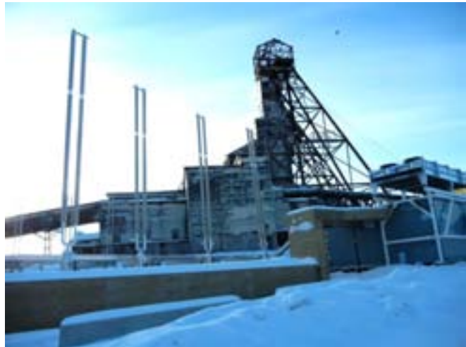
Thermosyphons at Giant Mine
