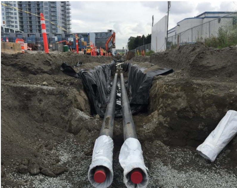
Figure 10: Buried Distribution Piping Installations
