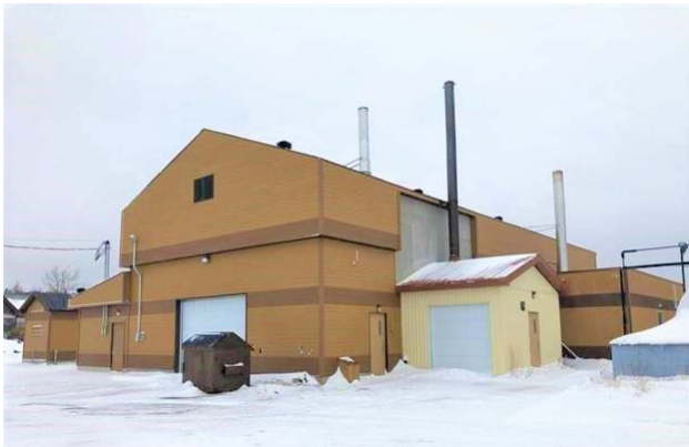
Figure 6: Oujé-Bougoumou Biomass Heating Plant
