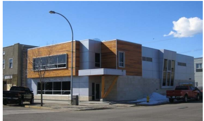
Figure 7: Prince George Downtown Energy Centre
